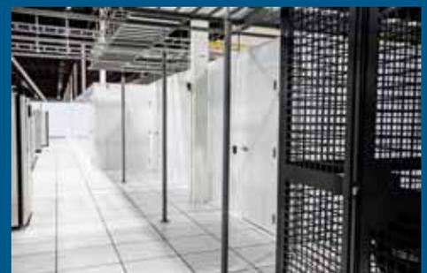
Walls can extend from floor to ceiling, allowing hot air to escape through the roof.
