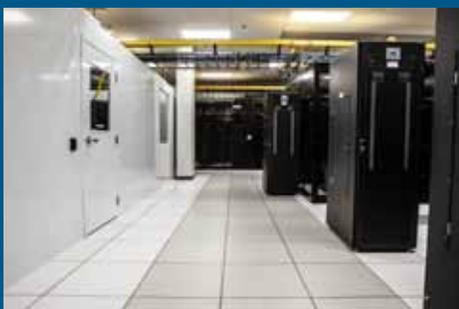
Hot and cold aisle configurations can be accommodated to funnel cool air into the server housing.
