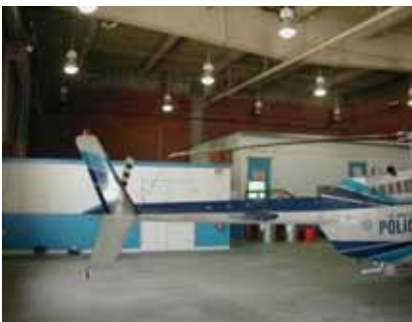
Training area prior to renovation
