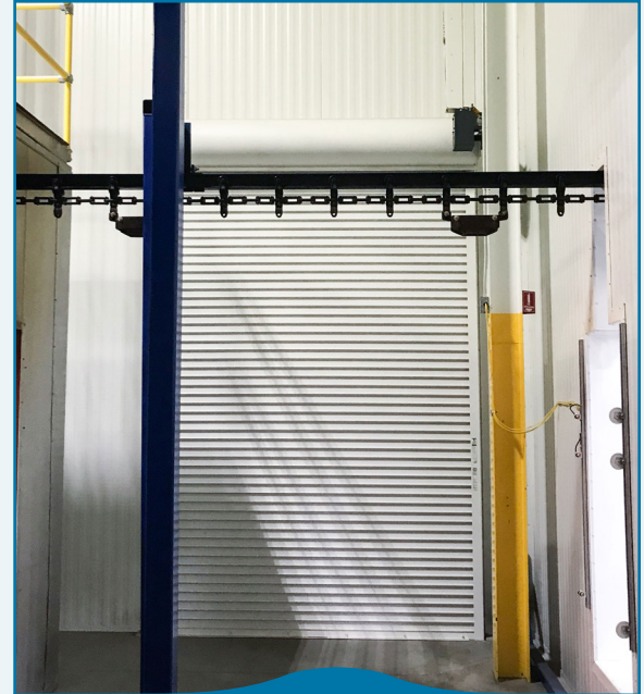
Overhead doors facilitate system maintenance and provide forklift access.
