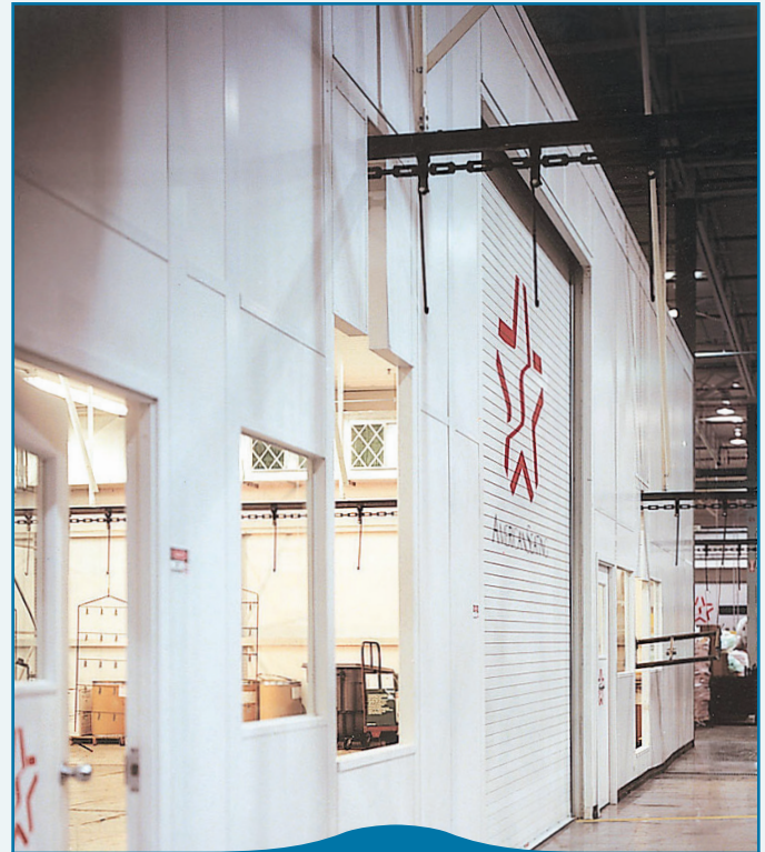
Keyhole conveyor opening
