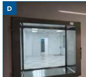
**D. Pass Through Chambers** - Pass through chambers minimize entry of contaminants by providing a means for pick-up and delivery of products and supplies without personnel entry. Productivity is increased while delivery personnel and contaminants remain outside.
