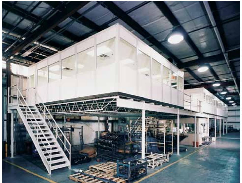
Offices on mezzanine give view of plant floor while allowing multiple uses of floor space underneath.
