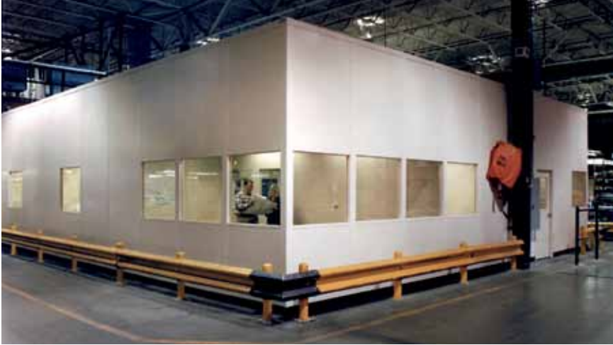
Office complex with protective guard rail.
