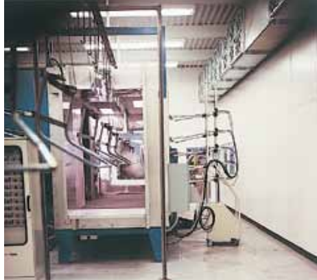
Powder coating application room.
