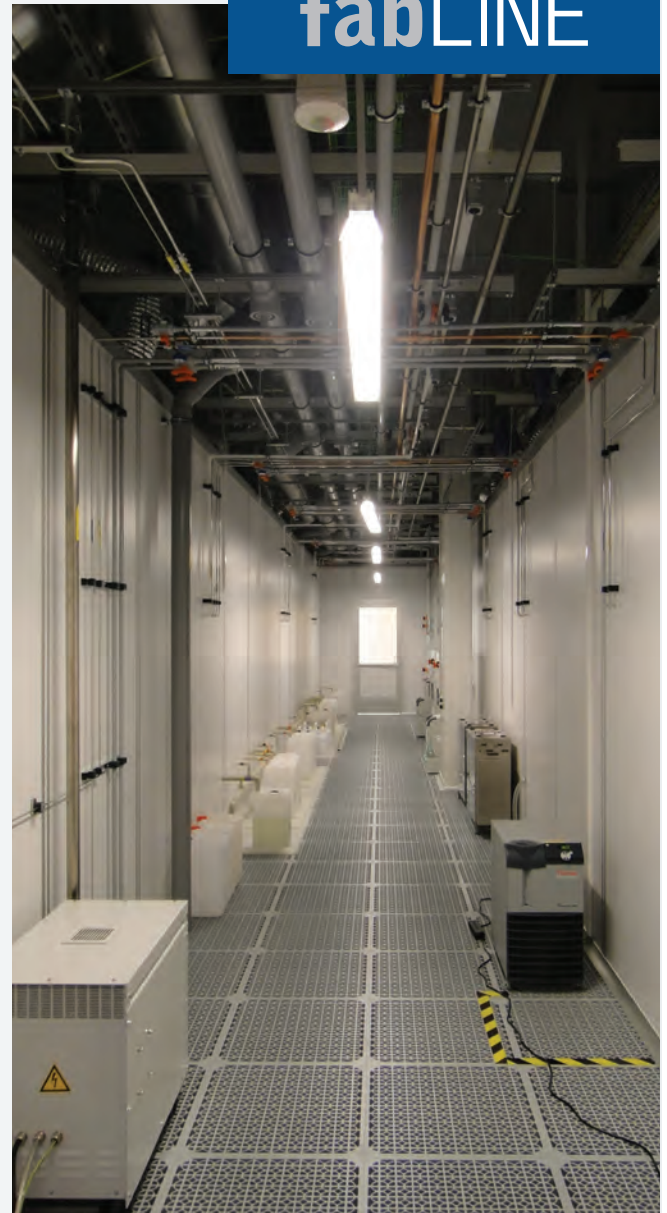
Chase side of a bay and chase Cleanroom featuring piping, conduit, and support equipment.
