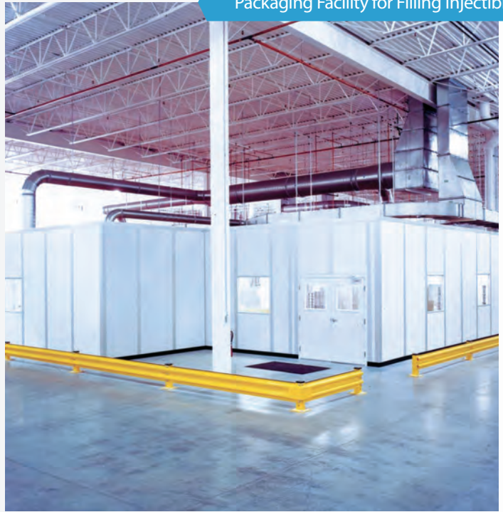
Packaging Facility for Filling Injectables
