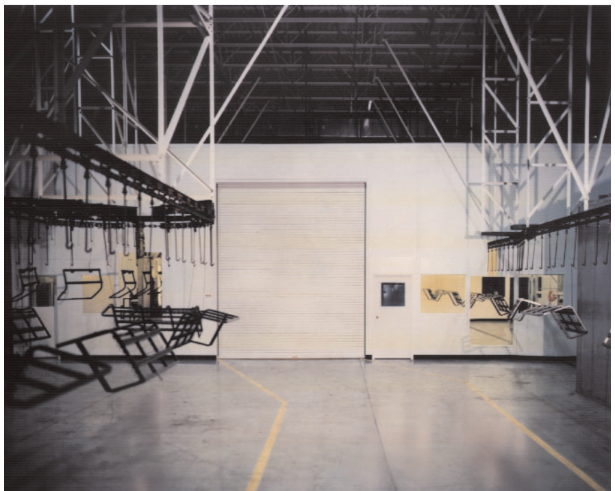
Overhead doors facilitate system maintenance and provide forklift access.
