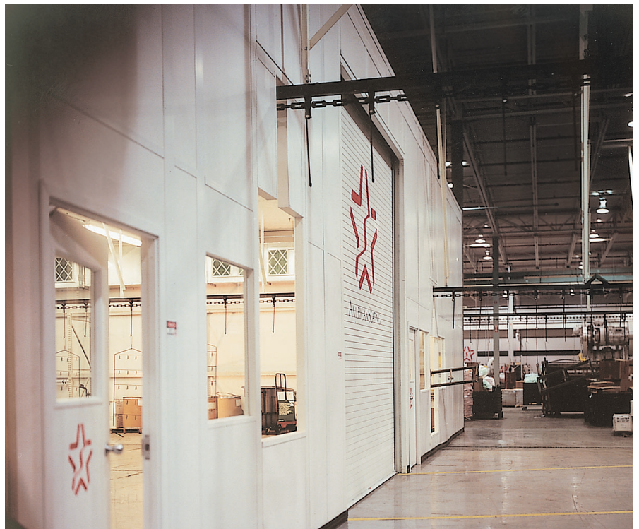
Keyhole conveyor opening.
