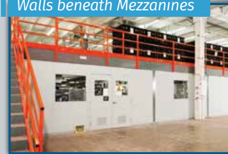
Walls beneath Mezzanines
