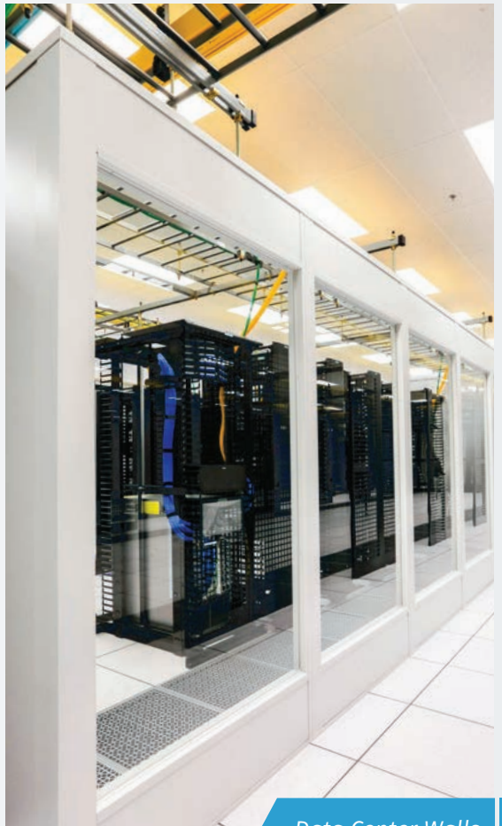
Data Center Walls
