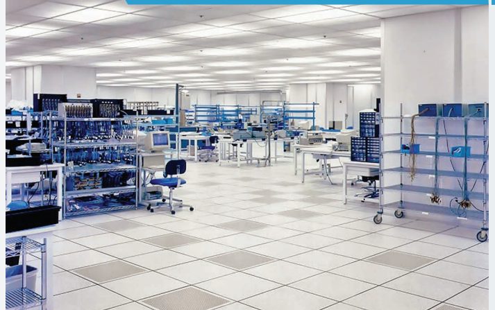
Electronics Cleanroom with Raised Floors
