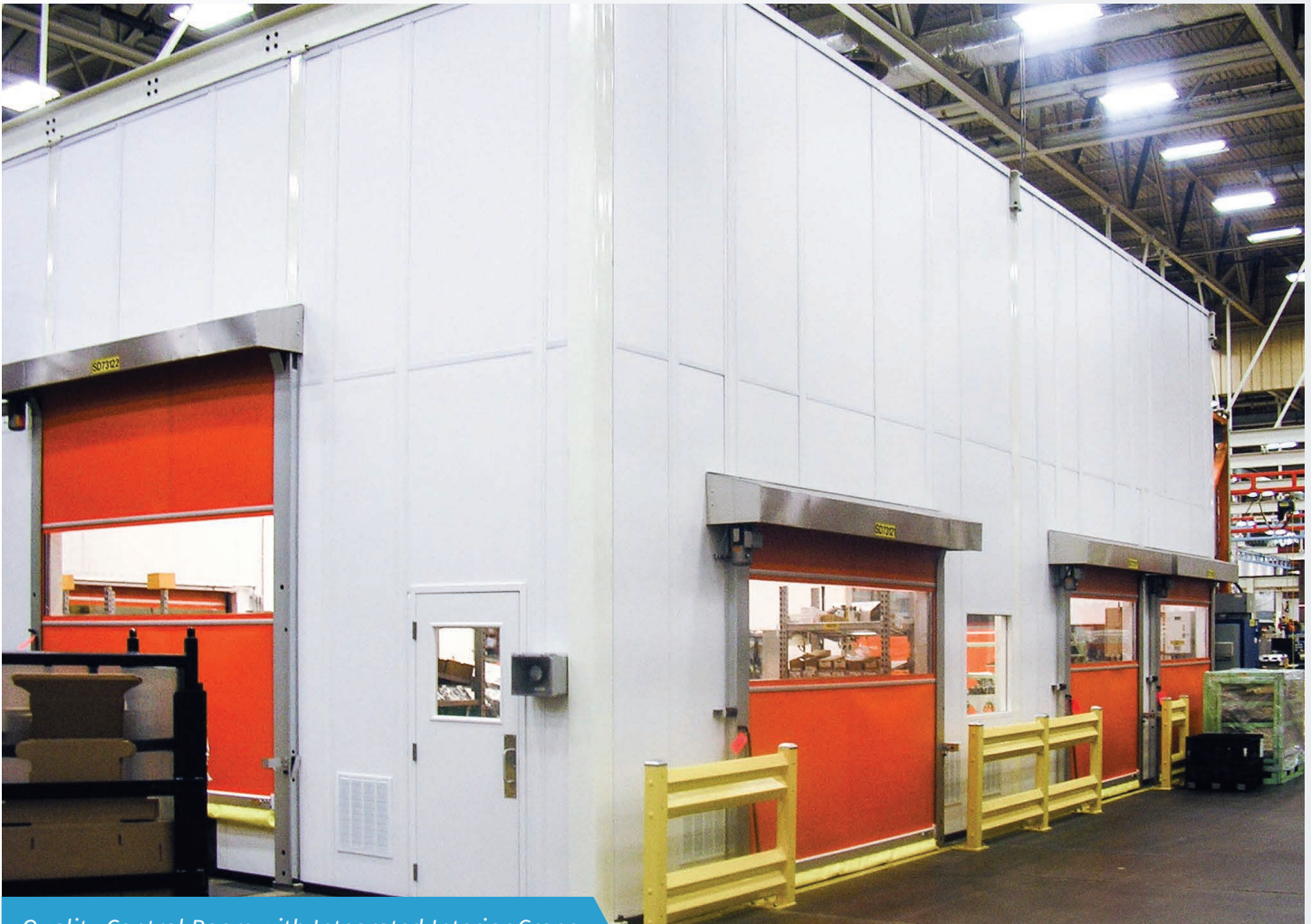
Quality Control Room with Integrated Interior Crane
