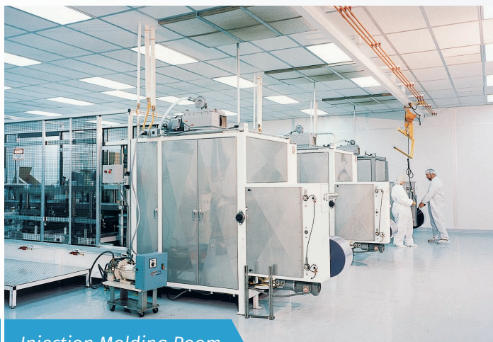
Injection Molding Room
