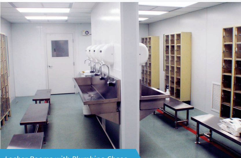
Locker Rooms with Plumbing Chase
